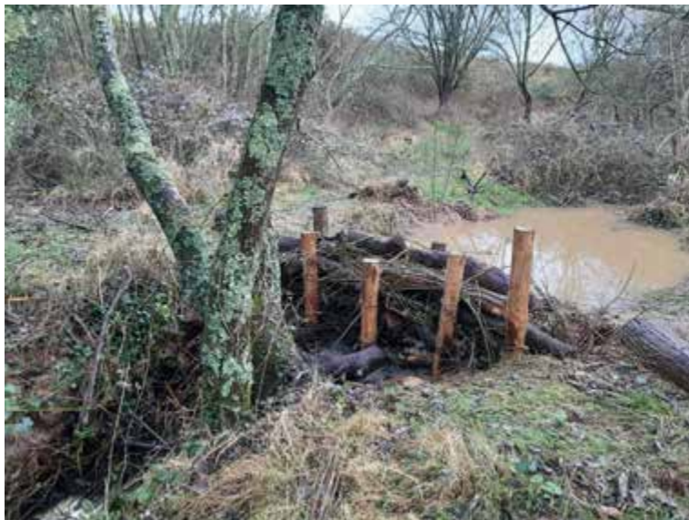
Leaky dam on Corfe Common, by Gen Crisford
