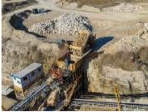
Suttle Stone Quarries' stone crusher at Swanworth Quarry, powered by electricity generated by on-site solar panels
