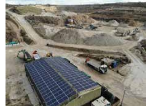
Solar Panels installed at Suttle Stone Quarries' Swanworth Quarry workshop.
